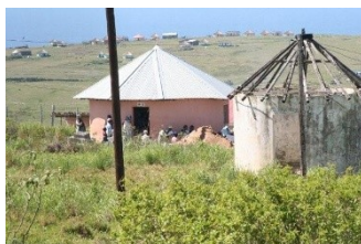
One of the huts before renovation...
