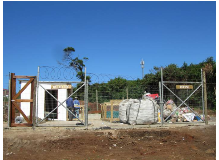
The centre under construction
