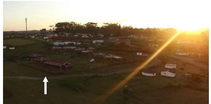
New houses at New Lundi
